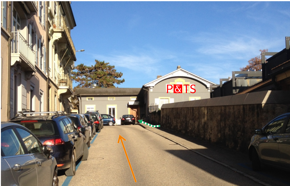
Go round the back of the Hôtel du Peyrou, the P&TS building is just above it.
